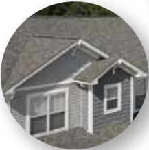
Roofing and Ventilation
